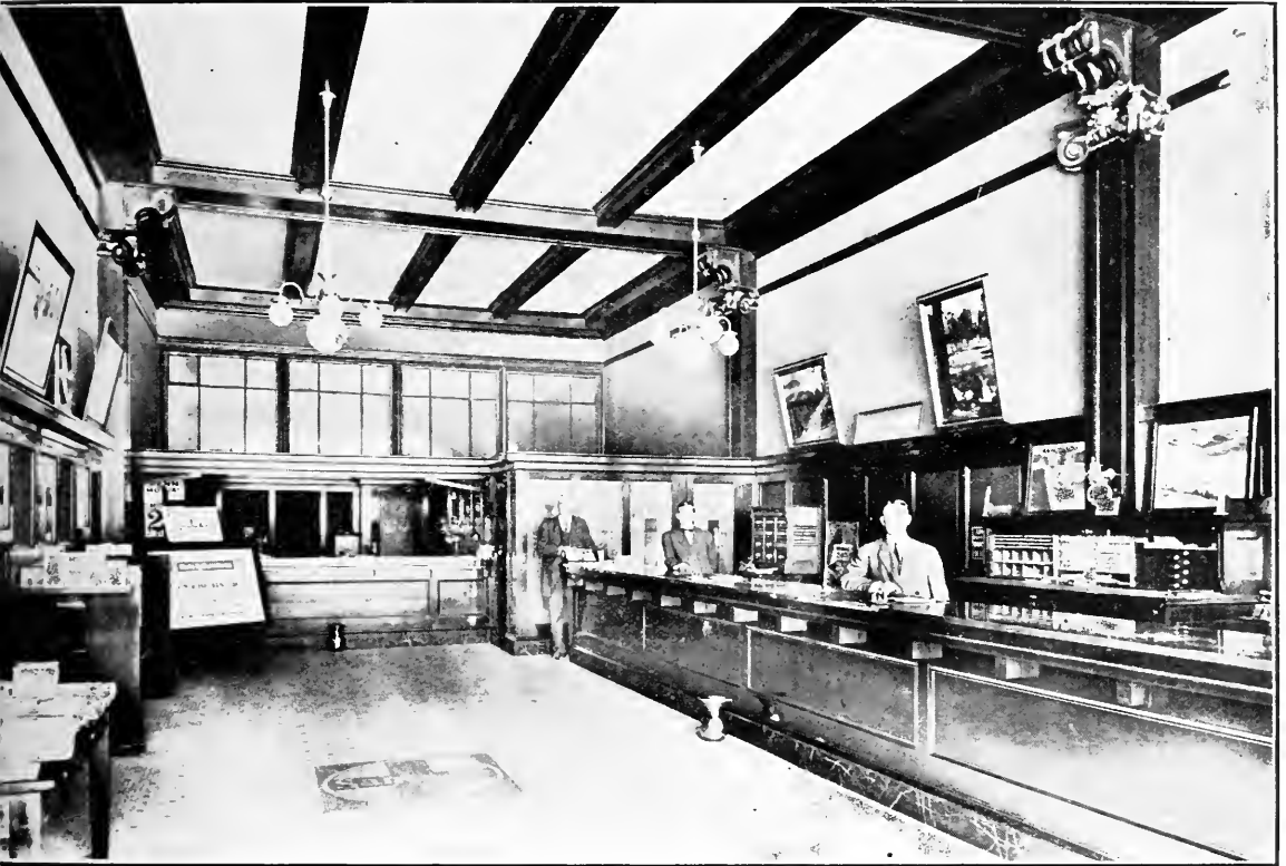
Interior Santa Fe Ticket Office, Oakland
